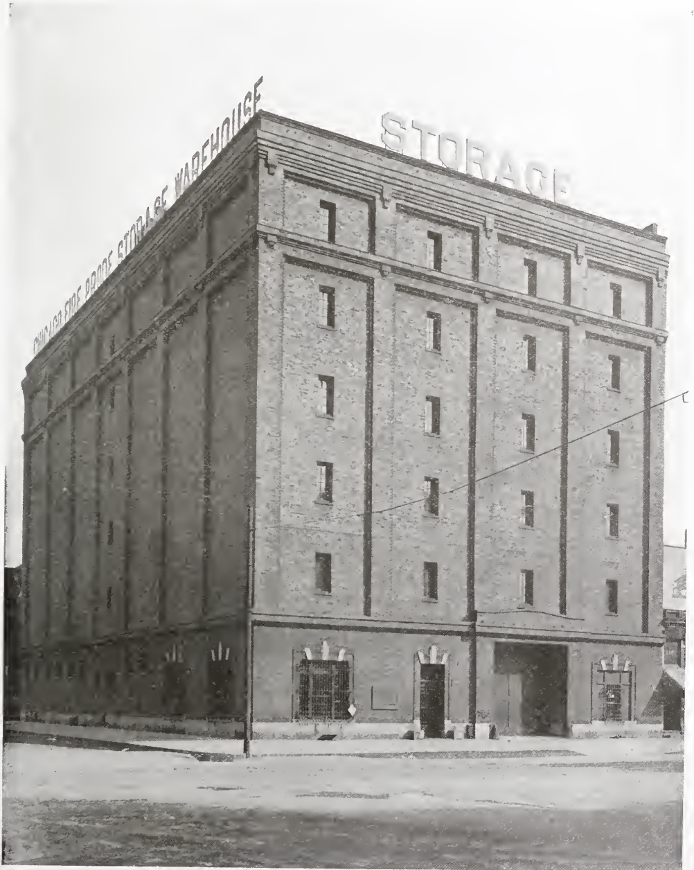
FIG. 7. THE CHICAGO FIREPROOF STORAGE WAREHOUSE.
